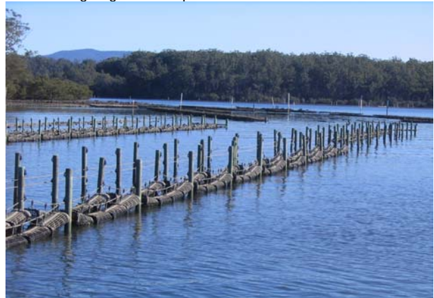
Conversion to plastic- 1/2ha trial of environmentally sustainable cultivation infrastructure
